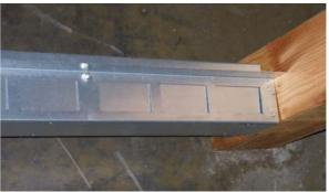
Figure 6-7: Fixing profile with slider (closed)
