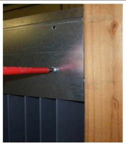
Figure 6-20: Fastening the back panels with tapping screws 5.5 x 13
