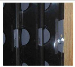
Figure 6-27: Fastening to the wooden post
