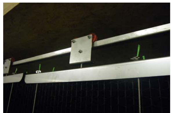
Fig. 13: Upper U-shaped profile with suspension ropes
