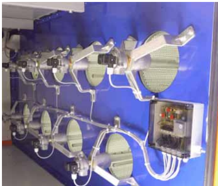
Figure 3-4: Positioning of the solenoid valves (clean gas side => 9 "Glossary")
